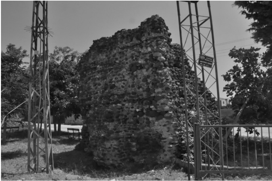
FIGURE 2.2 The Roman circus: concrete core of stairway 4
